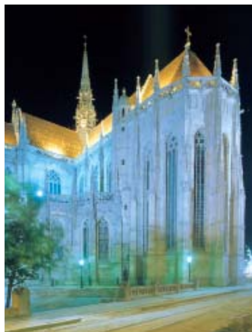
Saint Elizabeth's Dome in Košice
